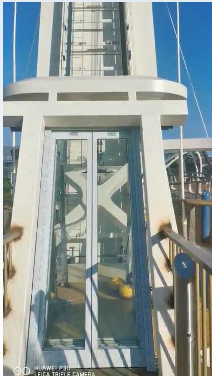
Hainan Sanya Duty-Free City Incline Lift Door Central opening 900*2100 glass doors Inclination Grade=30°
